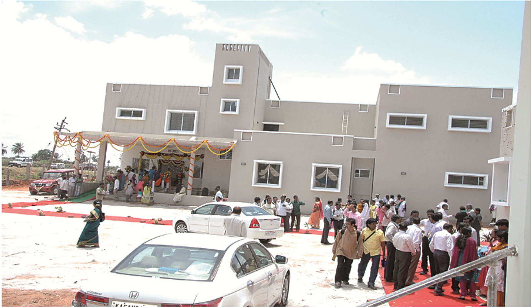
Administrative Block - Canara RSETI Chikbalapur, Karnataka
